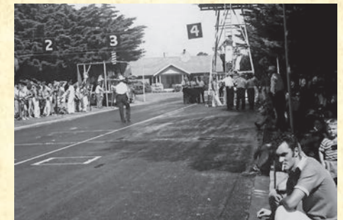
The competition track with the tower in full glory. That is Holcomb House on the Esplanade in the background.
